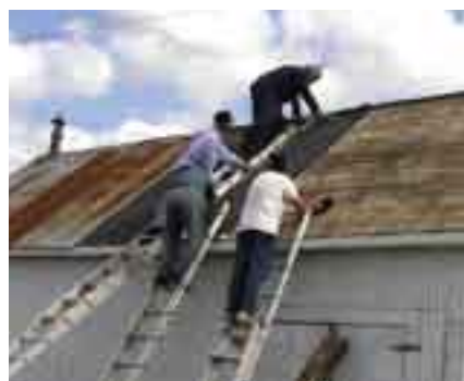
The 'work gang' installs a membrane on the roof. From top: Georges Jobin (consultant builder), Pierre Huberdeau, 'Foreman' Raymond Theroux and John Quayle.
