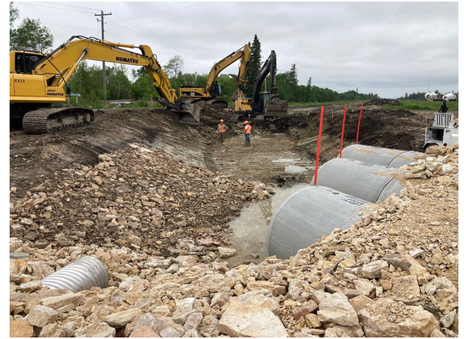
Grading & Culvert Replacement PTH 6 at Grahamdale
