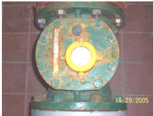
Photo 15: Distribution Water Meter
