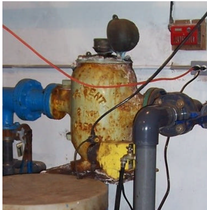
Photo 13 - Backwash Water Meter
