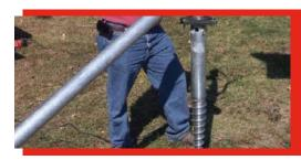
Our ground screw foundations use the natural compression of the earth for strength and stability.
