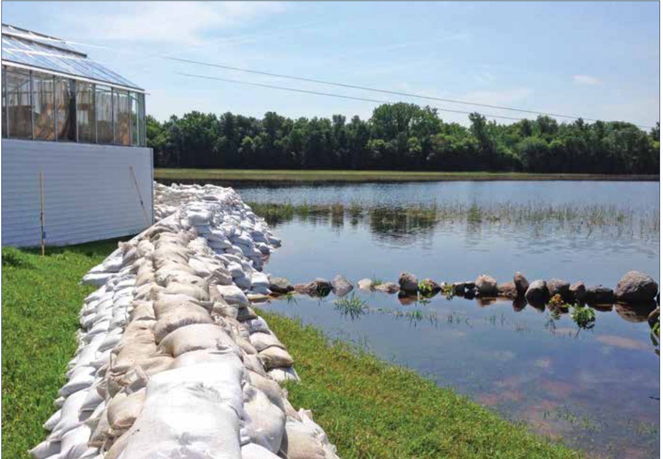
Photo by Jody Gale, emergency volunteer, along Hwy. 26 downstream of the Baie St. Paul Bridge. In early July, this house, 500 metres from the Assiniboine River, bordered a verdant field. After hours of work by army and volunteers placing 12,000 sandbags, this was the house on July 16.
