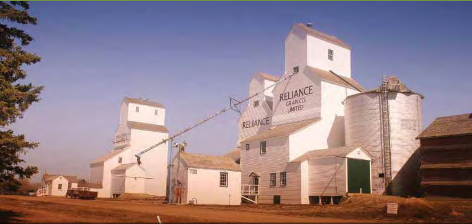
Looking north with the Reliance Double Elevators in the foreground and the Paterson Elevator and Visitor Centre in the background
