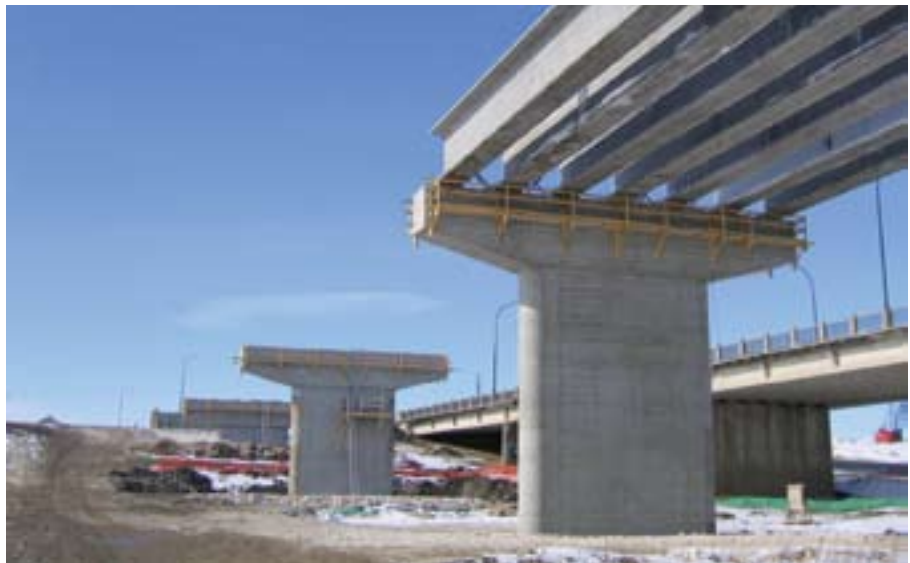
Girder Placement on Hwy. 1 East.
