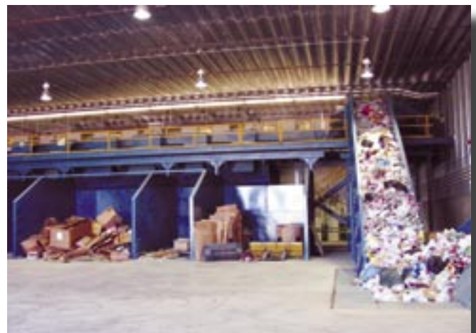
One-year-old, $4 million Westman Recycling Centre.
