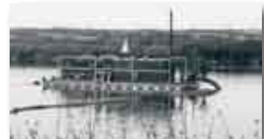
Roy & Sons Dredging Services have the "Solution"
